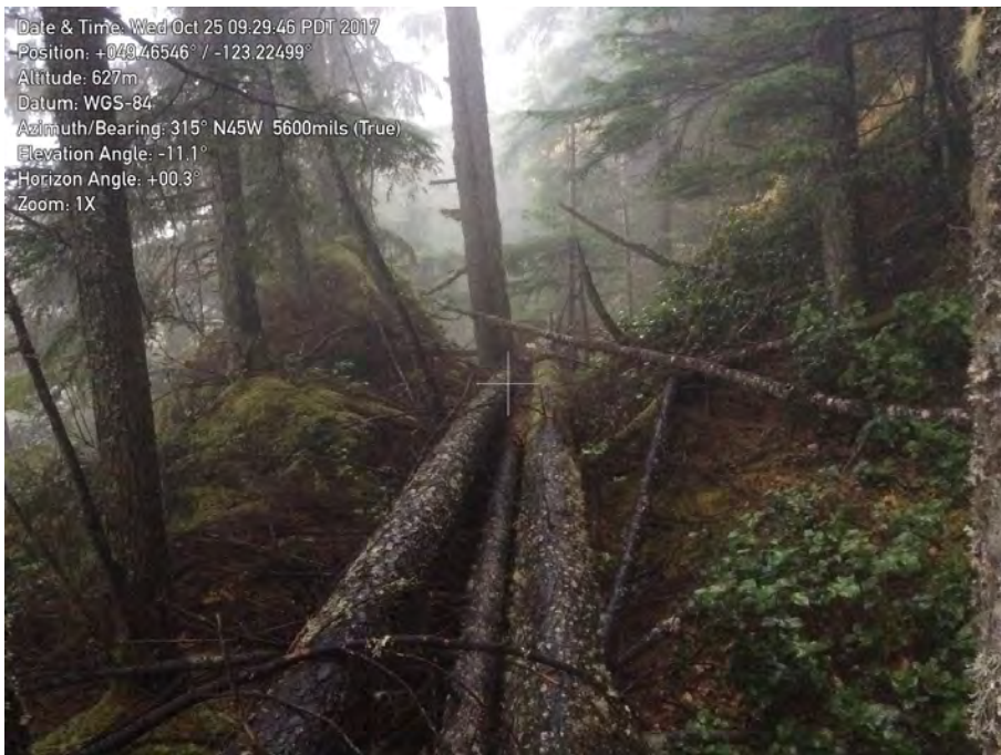
Photo 10. Waypoint 46. Antislope ridge indicating steep joint cutting crest of cliff. Several 10s m 3 to 1000s m 3 could be released from this site.
