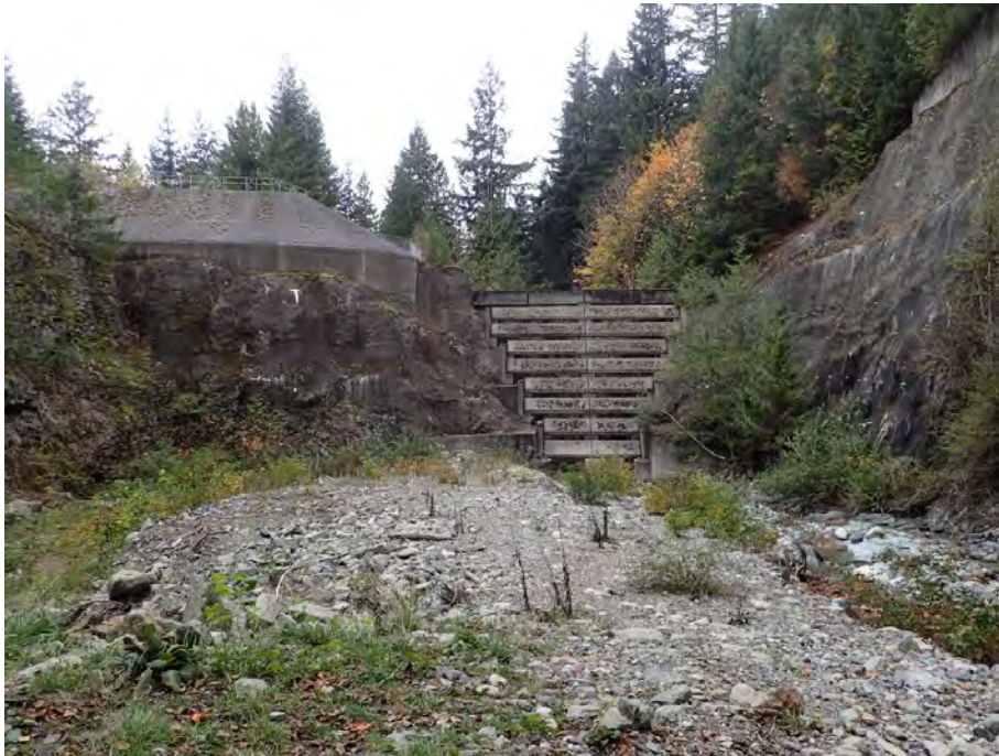
Photo 5. Magnesia Creek catch basin.
