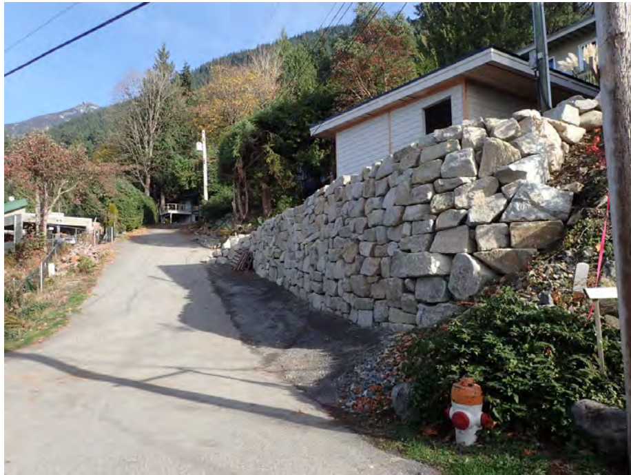
Photo 14. Lot 8 Islevue Place. Retaining walls in steep terrain require engineered design.
