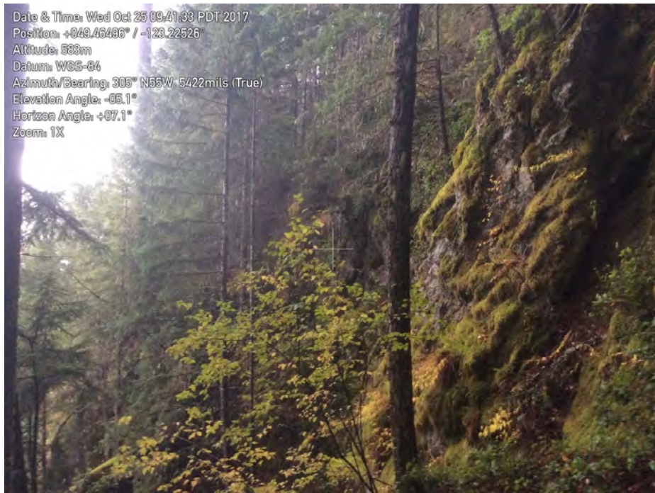
Photo 11. Bluff above Mountain Drive with unfavourable joint, parallel to steep slope.
