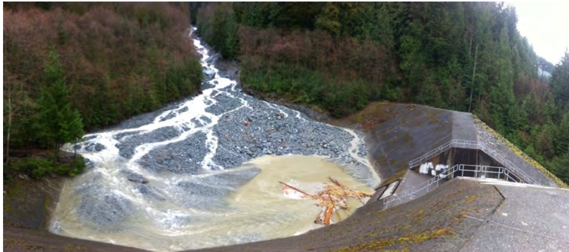
Figure 3. Charles Creek retention structure with debris flow inflow. Downloaded from internet ( https://www.flickr.com/photos/tranbc/8510095573 ).
