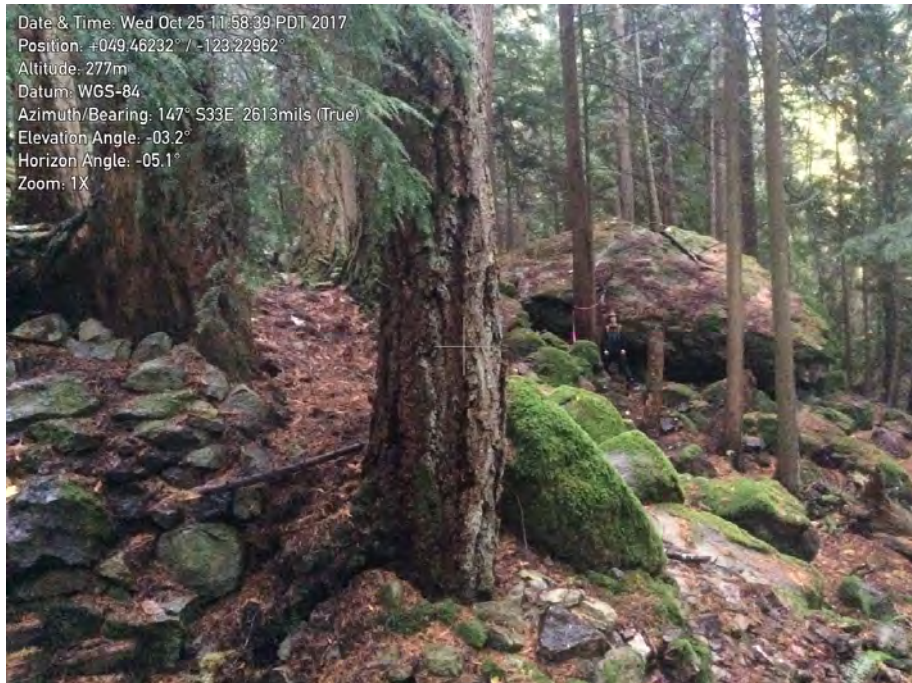
Photo 12. Rockfall debris, Lots A & B Timbertop Road. Note the person for scale.
